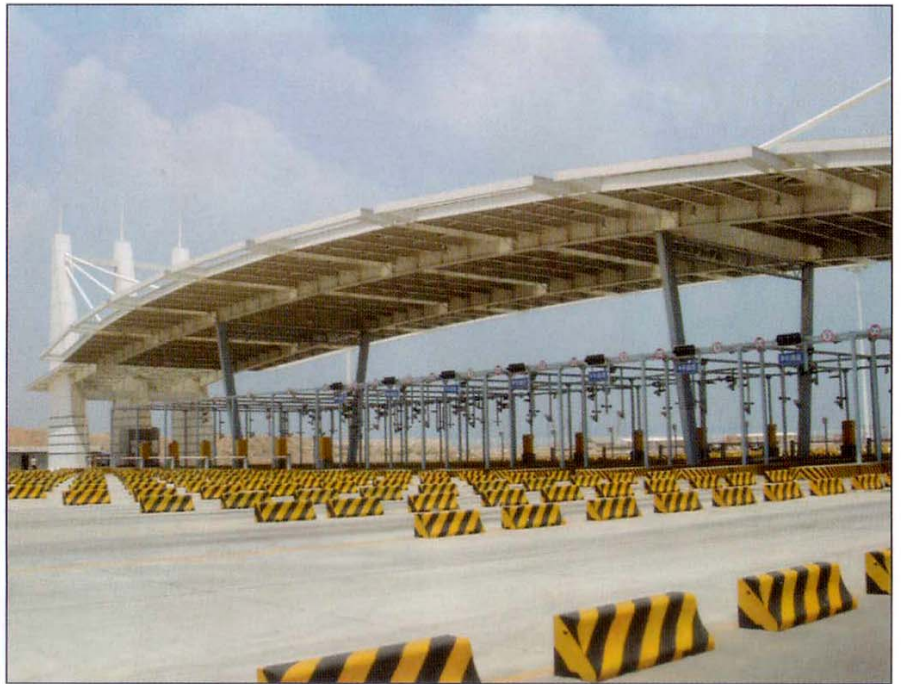
The new gate at Dalian Dayowan Phase II
